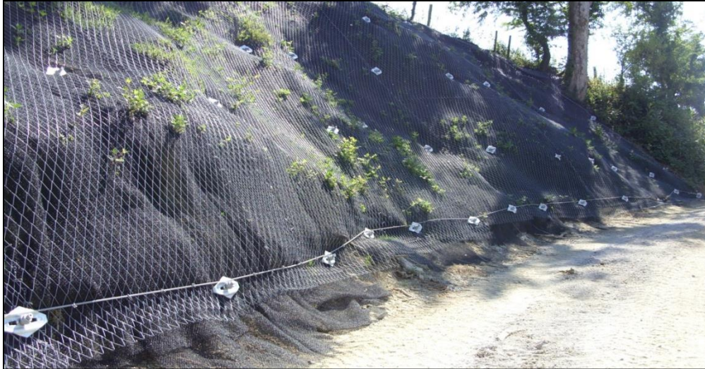
Soil nails at Beaminster Tunnel
